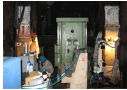
Fig.11: Field remanufacturing rolling mill framework.
