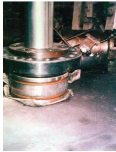
Repairing of abrasion of hydraulic pressure machine's column by adhesive
