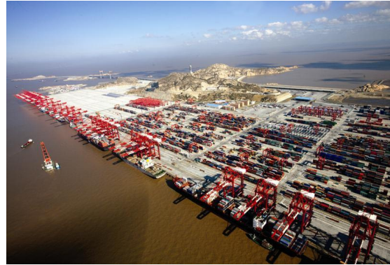
Figure 1.0-1 Yangshan Deepwater Port project
