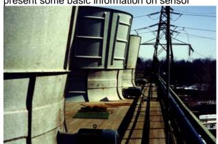
usage and placement for monitoring fans, motors and gearboxes on cooling towers.
