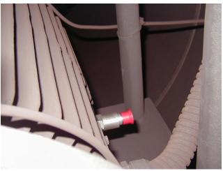
Horizontal Vibration Sensor Mounted on Tunnel Fan Motor
