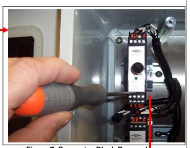
Figure 7. Connector Block Removal
