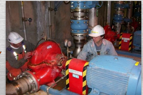
Execute Corrective Actions
