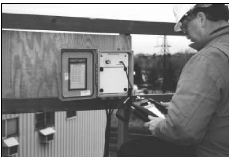
Figures 10 - Accessing data from switch box.
