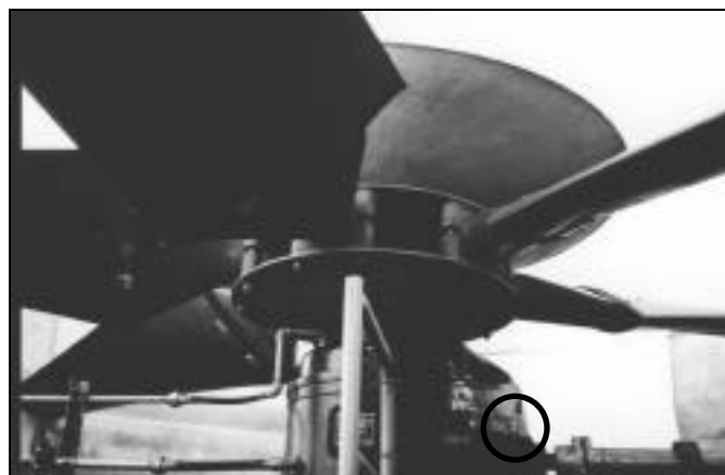
Figures 8, 9 - Permanently mounted accelerometers.
